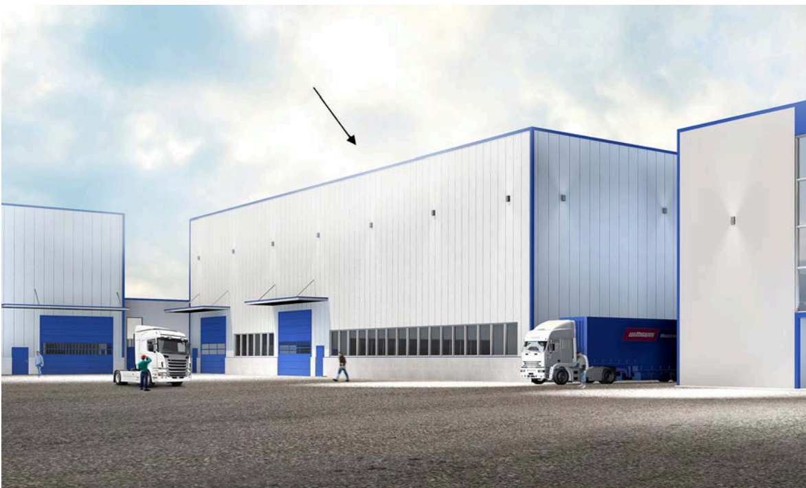
Fig. 2: Extension to the existing assembly hall in Kottlingbrunn – space: 3,000 m 2
